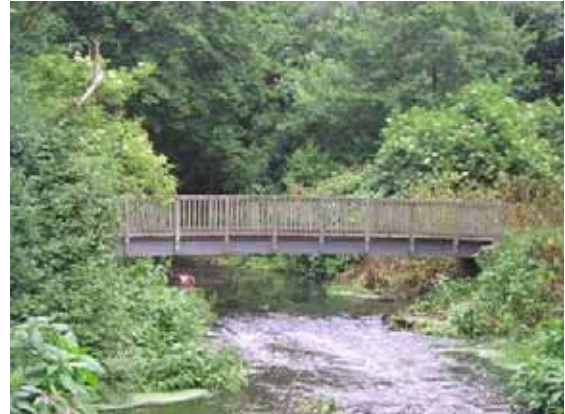
Figure 14: Mill Race Footbridge
