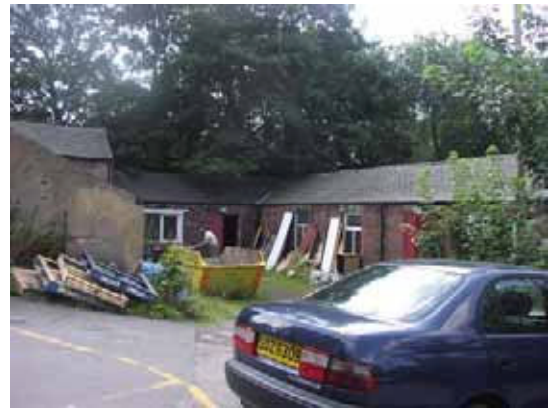
Figure 5: Courtyard Buildings (Units 16, 17, 18, 19 and 20)
