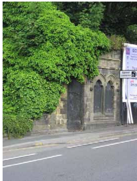
Figure 18: Remains of Former Police Building
