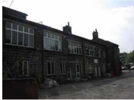
Figure 4: Abbey Road Buildings (Units 12, 13, 14, and 15)
