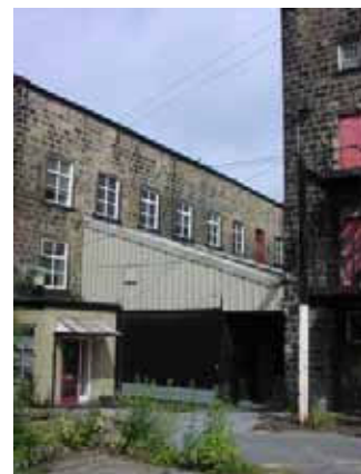
Figure 6: Modern Extensions Between Main Mill Buildings (Unit 7)
